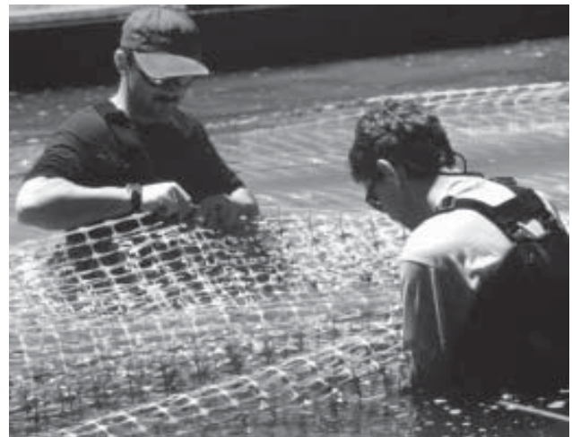
Figure 26. Substrate should be tied firmly to posts using 5 cable ties on each post. Posts should be about 45' apart.
